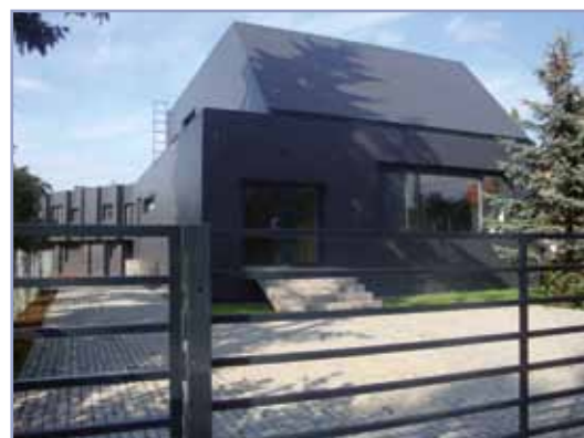
Hager Polonia Corporate Office Wrocław (Breslau), Poland
