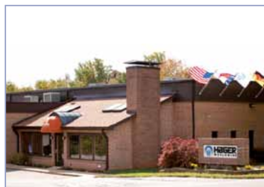
Hager Worldwide Corporate Office Hickory, North Carolina
